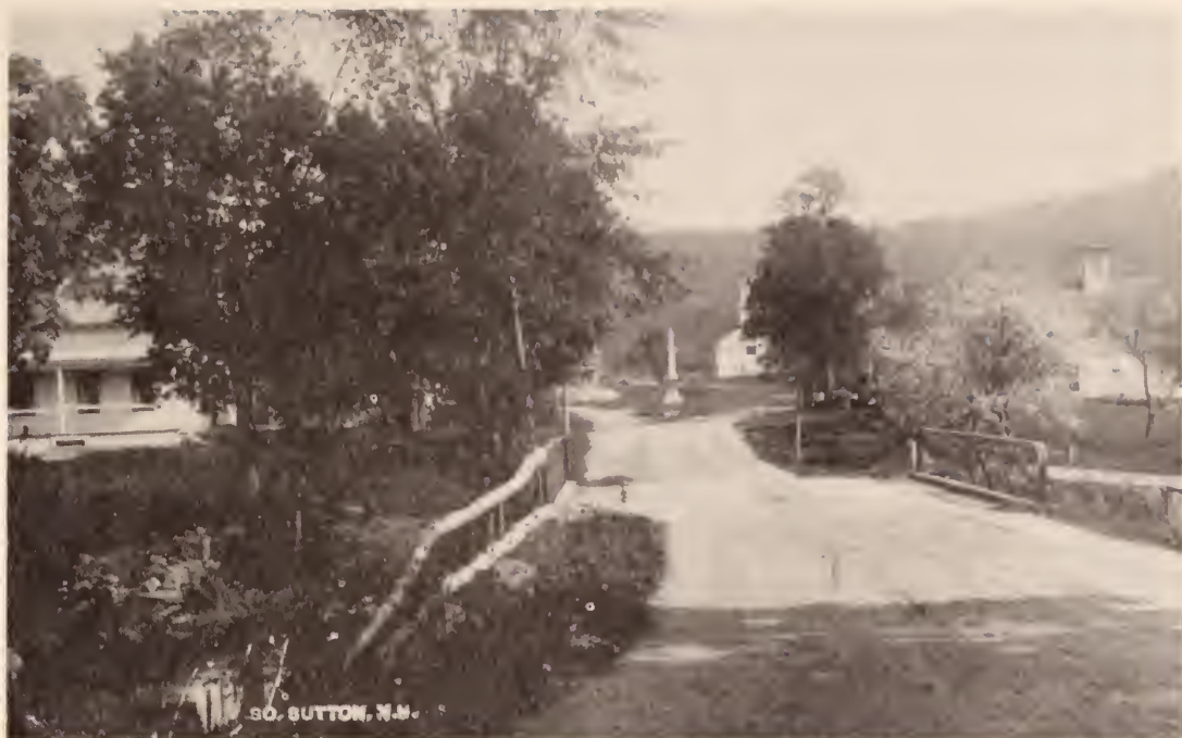
View of South Sutton, c. 1910, showing bridge over Lane River.
